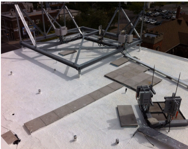
Cell Tower Roof
