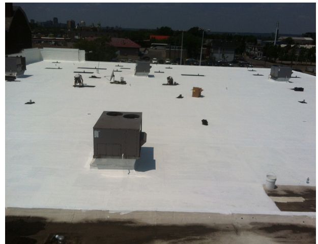
Grocery Store Roof
