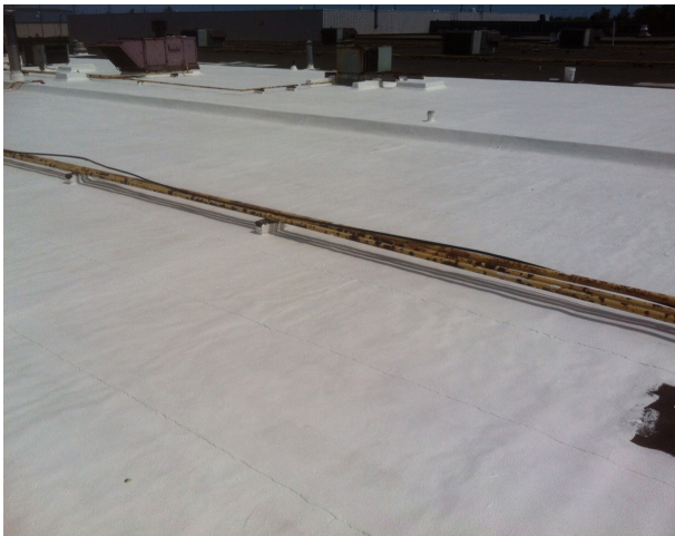
Strip Mall Roof
