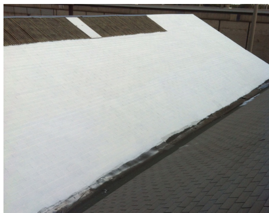
Roof Coat Over Shingles
