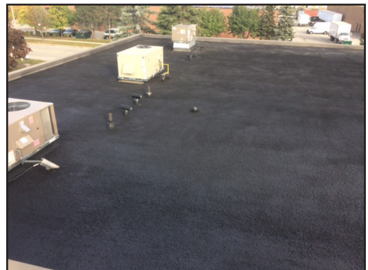
GRAVEL ROOF APPLICATION
